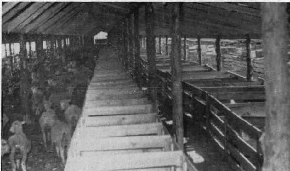
Interior of a modern lambing shed. Note that there are no sides on the shed so that sunlight can reach the center pen at some time of the day. Canvas walls are put up for protection during bad weather.
